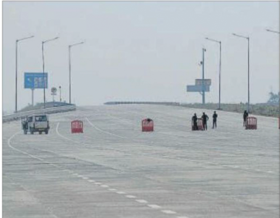
The Delhi-Mumbai Expressway near Hilalpur toll plaza after its inauguration. PARVEEN KUMAR/ HT PHOTO
